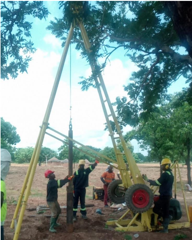
Caption: Percussion drilling onsite
