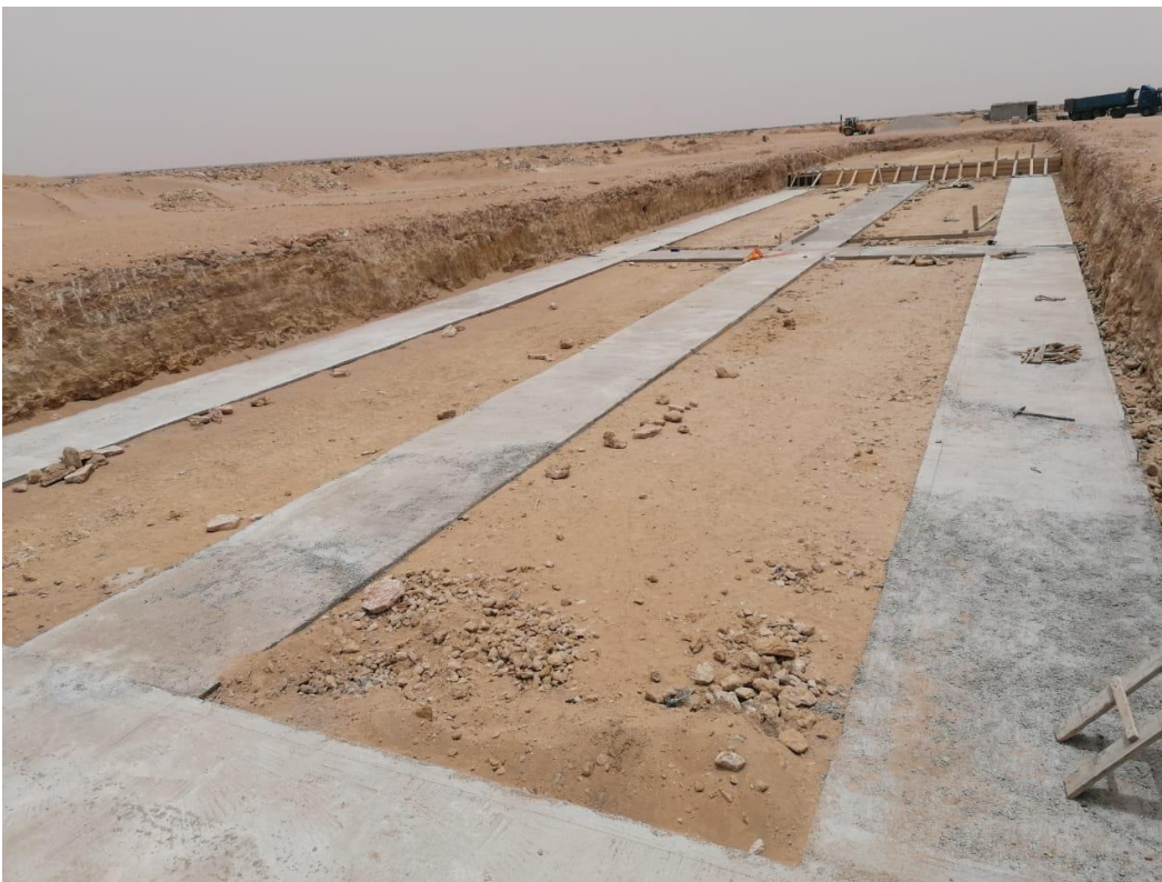
Caption: Concrete works in progress
