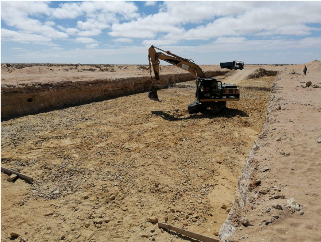
Caption: Tarfaya Wastewater Treatment Plant earthworks
