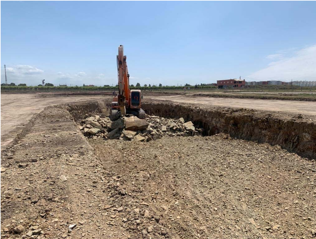
Caption: Bouznika Wastewater Treatment Plant earthworks
