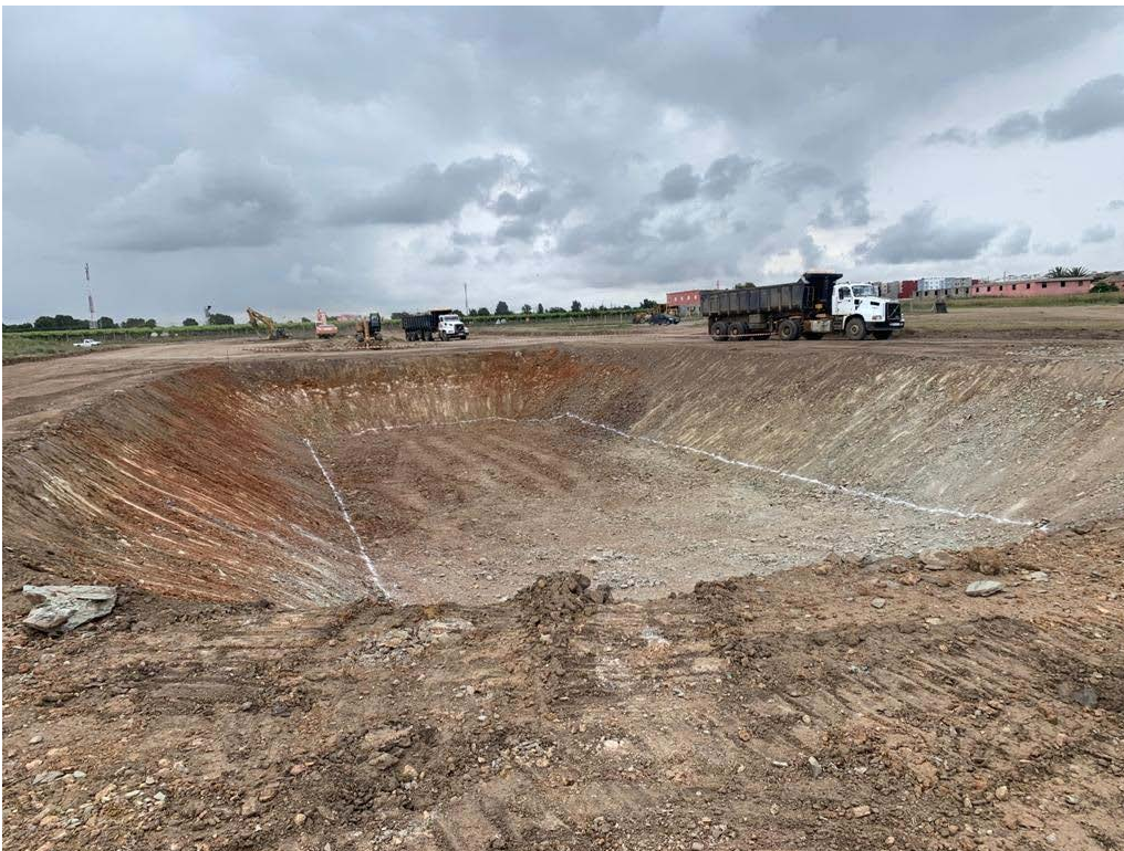
Caption: Bouznika Wastewater Treatment Plant earthworks
